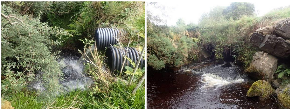
Plate 26: Site 8 on the Killuran Stream (left). This perched culvert represents an impassable barrier to upstream fish migration. Existing internal track crossing of the Coumnagun Stream (right). Brown Trout occur upstream of this location.
