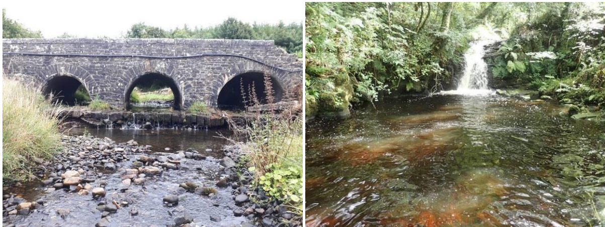
Plate 16: Bridge plinth on the Killuran Stream at Site 7 represents an upstream migration barrier for some species including lamprey and perhaps European eel (left). Waterfall on the Killuran River upstream of Site 7 (right). Sudden river profile changes such as this limit upstream migration of fish into the proposed project site.
